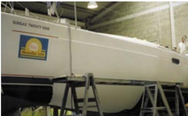
**4** Colour-matched white gel coat, built up behind with chopped strand mat, has been used on the repair. Once the mould has been removed, additional layers of colour-matched gel coat will be applied from the outside. These will be repeatedly applied and sanded back until the whole hull is fair.
